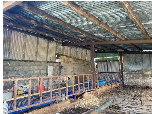
Plate 4-20 Internal view of Structure 2, a large farm shed constructed of brick and corrugated iron.
