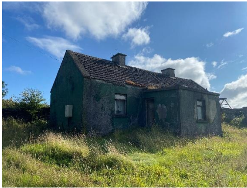
Plate 4-9 External view of the vacant single-storey house (Structure 8) showing intact slate roof and surroundings.
