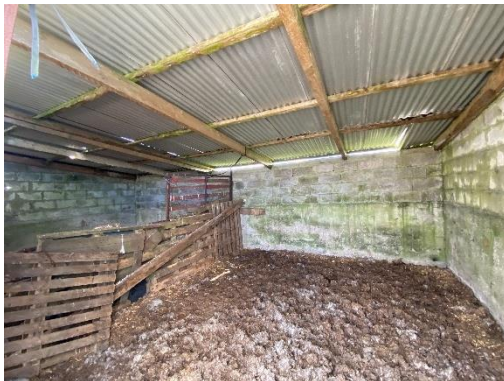
Plate 4-19 Internal view of Structure 1, a small cattle shed with corrugated iron roof.
