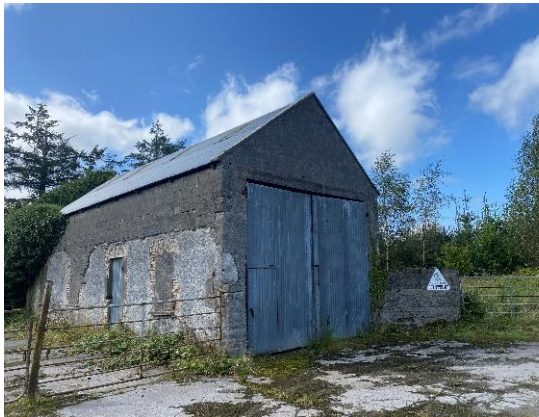
Plate 4-13 External view of Structure 3, with corrugated iron roofing, located southwest of Turbine 1.
