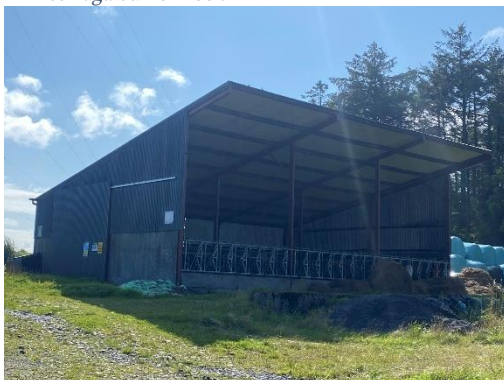
Plate 4-21 External view of Structure 4, a large modern cattle shed with surrounding trees.
