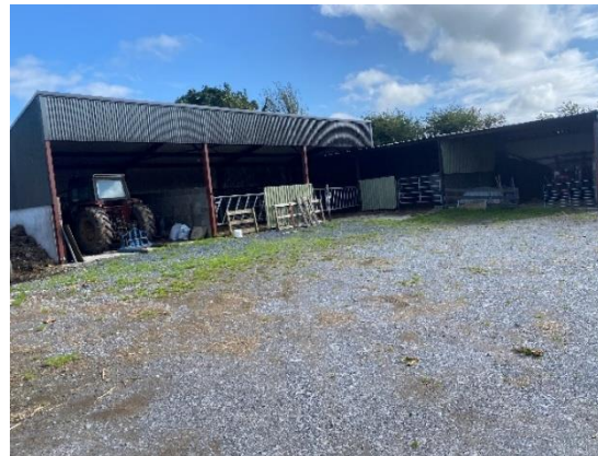
Plate 4-16 Corrugated iron sheds adjacent to the main building, currently in use as part of the active farm complex.
