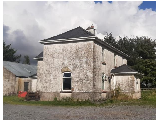
Plate 3-2 Western Face of the Dwelling
