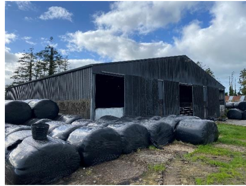
Plate 4-24 External view of Structure 11, a large metal agricultural shed.
