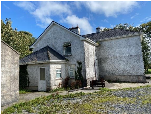
Plate 4-5 External view of the vacant farmhouse building showing intact slate roof and concrete-rendered exterior.
